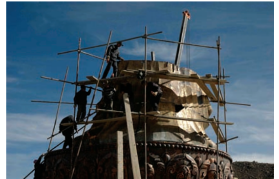
The statue of Guru Rinpoche under construction, pictured in February [ICT].
