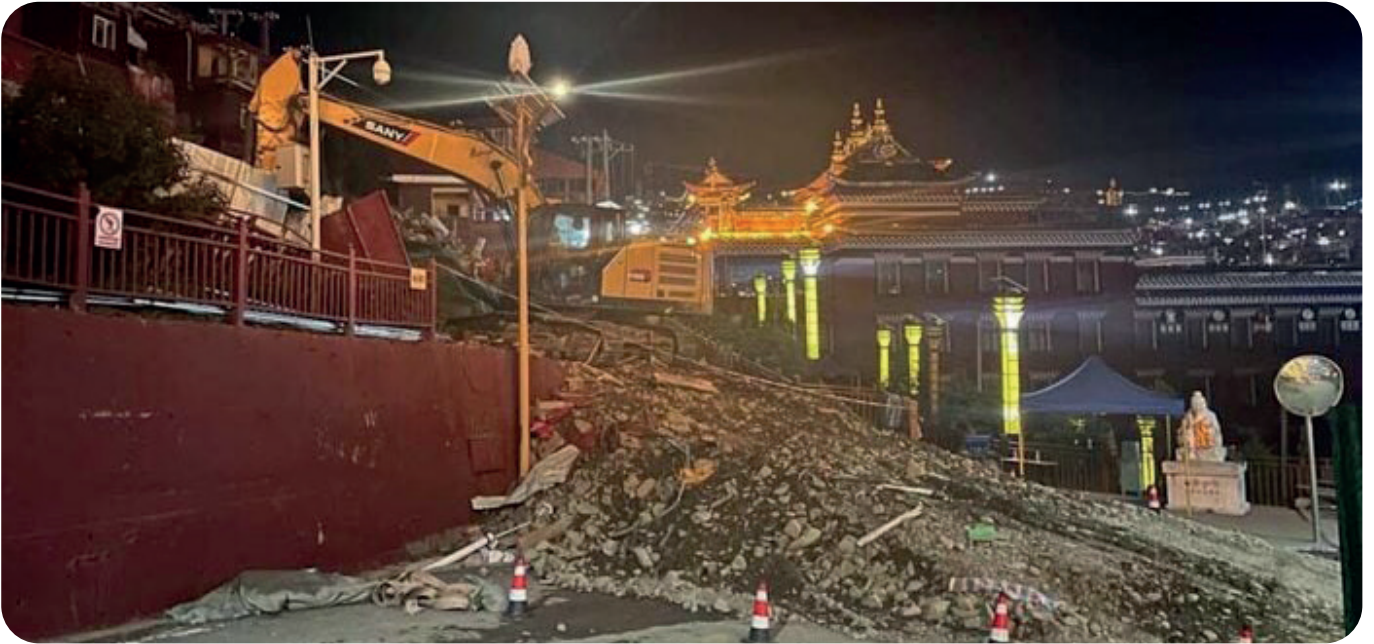
Another August 13-dated photograph shows proximity of the latest round of demolition work being carried out at Larung Gar to the center of the Buddhist academy. (ICT sources)
